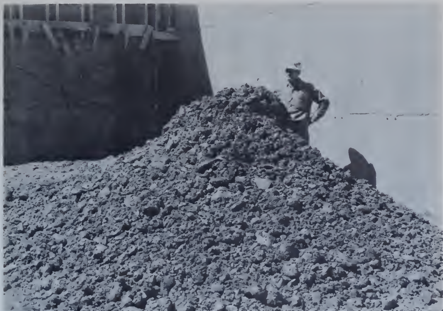
Figure 139.—Eight cubic yards of concrete immediately after being deposited. PX-D-25254.
